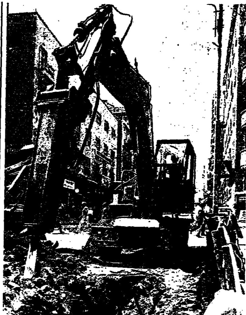
THE CROOKED ARM of a giant hydraulic hammer is used to dig up the peaceful pedestrian mall part of Ben-Yehuda Street in downtown Jerusalem to prepare for the laying of telephone lines. The machine is said to be the only one of its kind in the country. (Steve Nelson)
